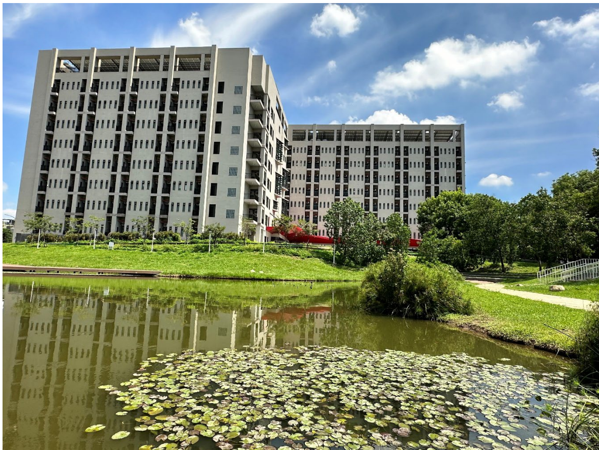
The Mingxiu Lake of NCUT can be used as an ecological lake at the campus, and it also has a function of detention ponds, which can regulate the amount of water.
